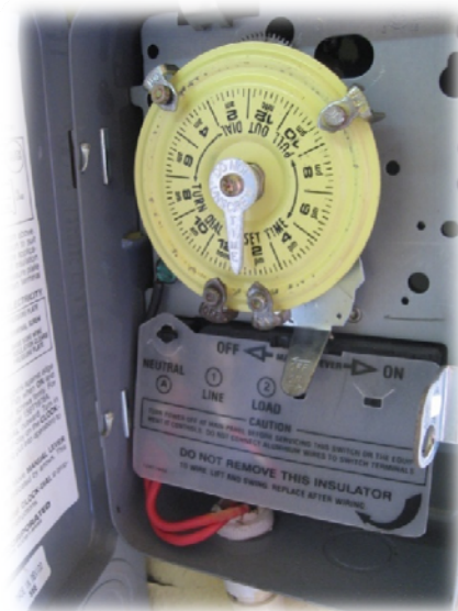
Figure 2.5-4 Independence Pump Supply Timer
