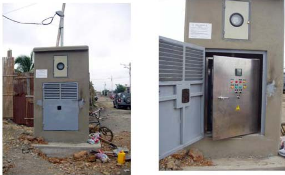
Outdoor Electrical Control Panel – Protected Against Vandalism
