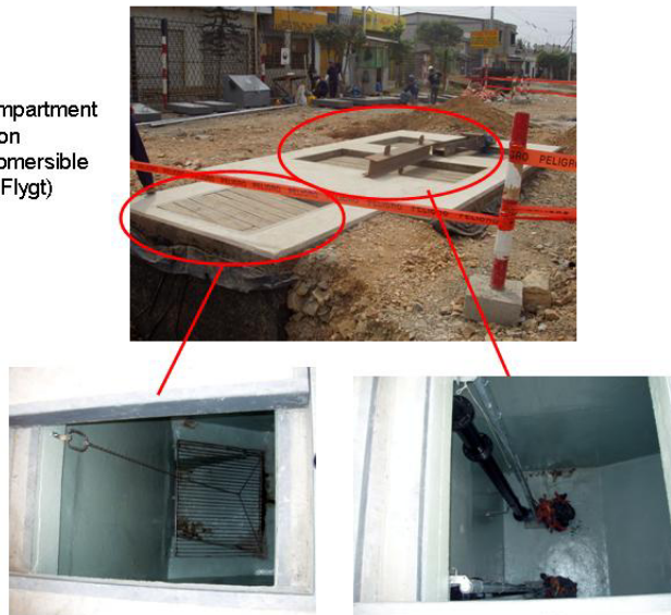
Figure 4.2-1 Submersible Pump Station
